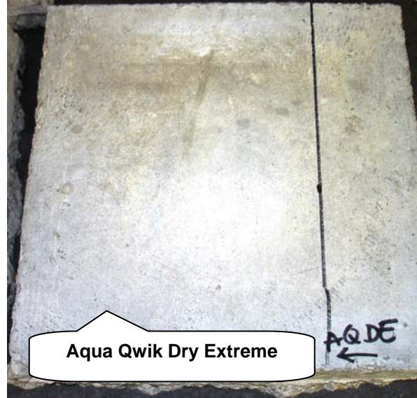
Steel Troweled Concrete After Stain Testing
